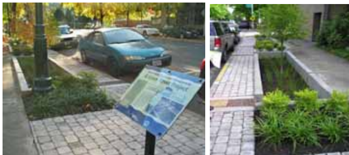
An example of a green street in Portland. Information signage highlights the sustainable elements of the street making the connection between the ecosystems, infrastructure, and the urban environment. Planters and permeable pavement provide habitat, slowly release storm water flow, filter pollutants and reduce erosion. Water management will be a key element of sustainable streets in the Downtown (Image from City of Portland).
