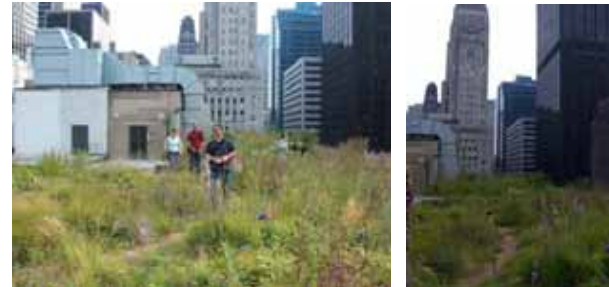
A Green Roof at Chicago's City Hall. Green Roofs improves aesthetics, removes carbon, improves building efficiencies, provides onsite storm water management and can offer greenspace for residents and workers.
