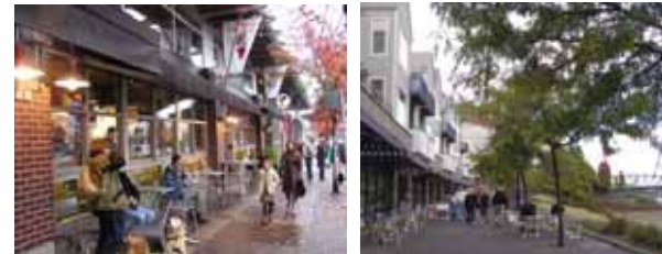
ABOVE: Overhead weather protection extends usability of the sidewalk seating areas and an active building frontage provides numerous points of interests and interaction.
