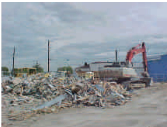
Demolition work moves ahead in the Fort Road area.
