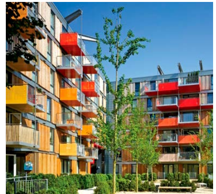
Figure 19 Medium Rise Apartments
