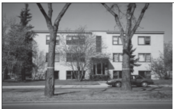
Typical older apartment
