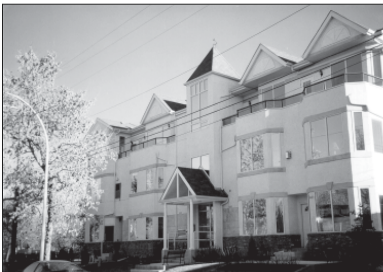
Front entrances, façade treatment and set back of the upper storey maintains street character
