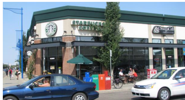
Building built to front and side property lines.
