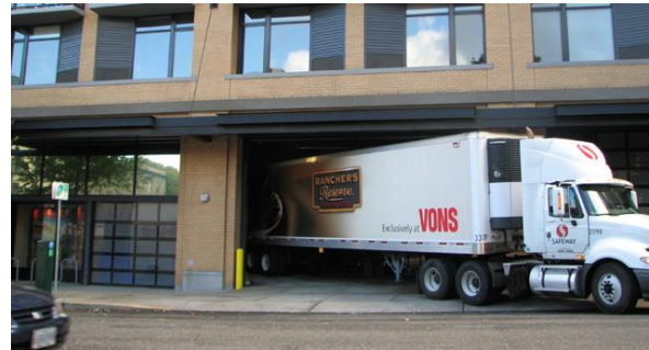
Truck backing into a fully enclosed loading dock designed to minimize its prominence.
