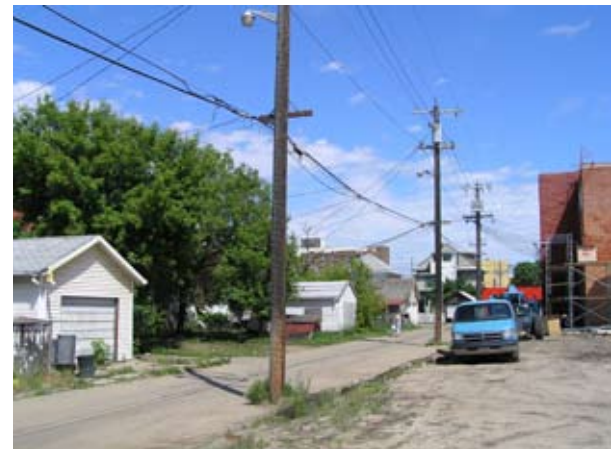
Existing utility services
