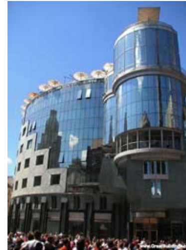
Curved and rounded building forms reflect the uncommon shape of blocks
