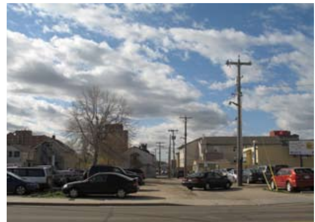
Overhead wires along laneway of 96 Street
