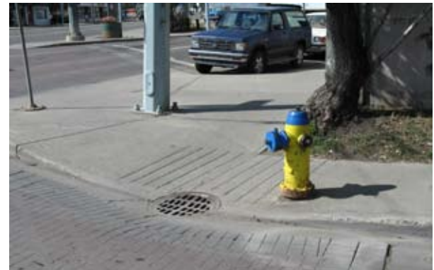
Existing utility services
