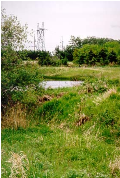
View of creek showing TransAlta right-of-way.
